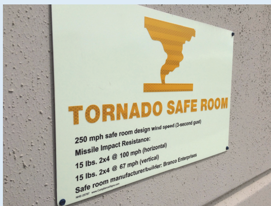
Figure 3-1 Tornado safe room placard.
