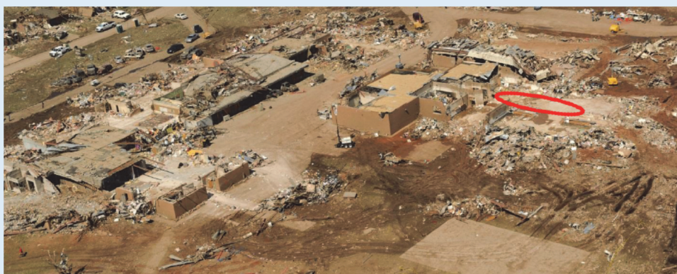
Figure TO-12 Post-tornado view. The area circled in red shows the approximate location in the hallway where the 7 fatalities occurred (NIST, 2013; Original photo source: NOAA).
