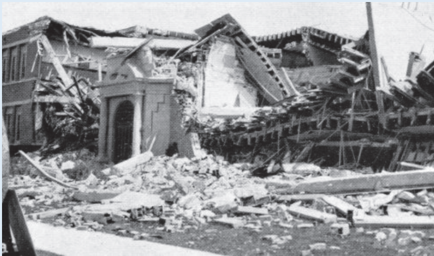
Figure E-4 Collapse of part of Jefferson High School in the 1933 Long Beach earthquake. (Photo source: Portland Cement Association)
