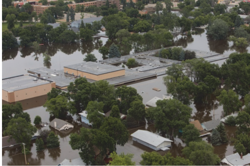
Figure F-1 Ramstad Middle School, in Minot, North Dakota was flooded in June 2011, badly damaged, and ultimately decommissioned in June 2012. A replacement school was constructed in a less floodprone area.
