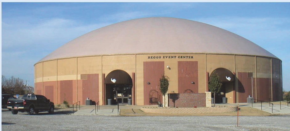
Figure 3-2 Thanks to a federal grant, a new monolithic dome resembling the existing Beggs Event Center (shown here) will house Beggs School District’s tornado safe room. (Photo source: Monolithic Dome Institute)
