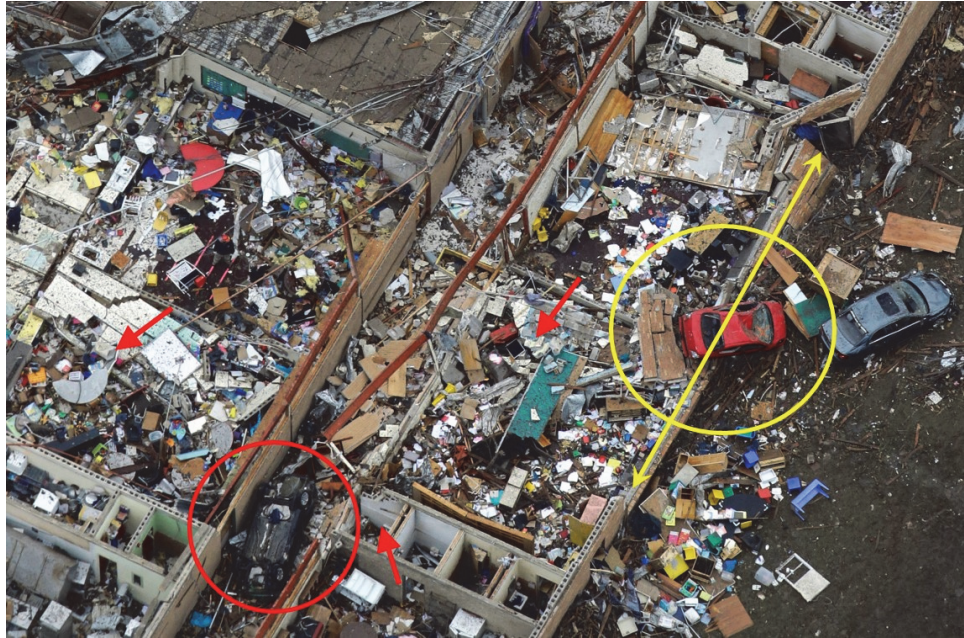
Figure TO-3 Aerial view of a school devastated by a strong tornado in Moore, Oklahoma in 2013 (Photo source: AP Images). Yellow circle indicates where a wind-blown car impacted an exterior wall (yellow line) and pushed it into a classroom. Red circle marks an upside down car in the hallway, and the red arrow indicates collapsed interior masonry walls.
