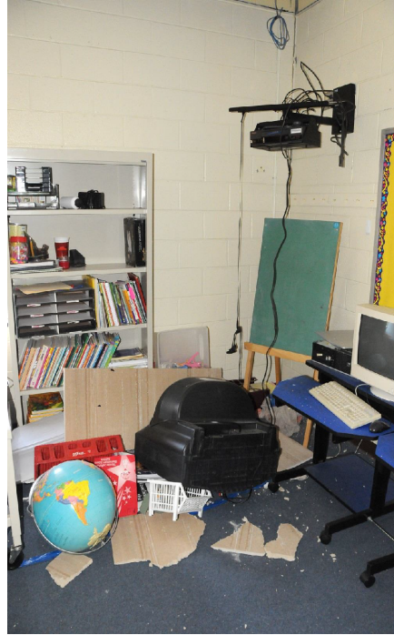
2011 5.8 M_w Mineral, Virginia earthquake. Fallen television in the classroom. (Pettit, 2014)
