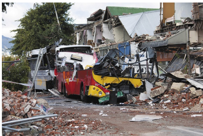
Left: City bus crushed by URM debris falling from nearby buildings during the 2011 Christchurch earthquake. Twelve of the 13 people on board were killed. Photo credit: Simon Baker 6 Right: Sidewalks, vehicles and portions of the roadway were buried by debris in downtown Christchurch during the 2011 earthquake. Photo credit: The Press/Fairfax NZ 7
