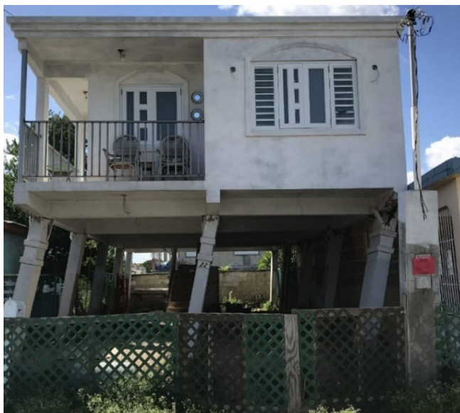
Red placarded 'unsafe' home leaning precariously over an undamaged adjacent home after the 2020 Puerto Rico earthquake. Photo credit: FEMA
