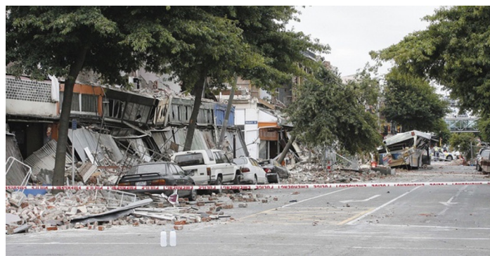
Left: City bus crushed by URM debris falling from nearby buildings during the 2011 Christchurch earthquake. Twelve of the 13 people on board were killed. Photo credit: Simon Baker 6 Right: Sidewalks, vehicles and portions of the roadway were buried by debris in downtown Christchurch during the 2011 earthquake. Photo credit: The Press/Fairfax NZ 7
