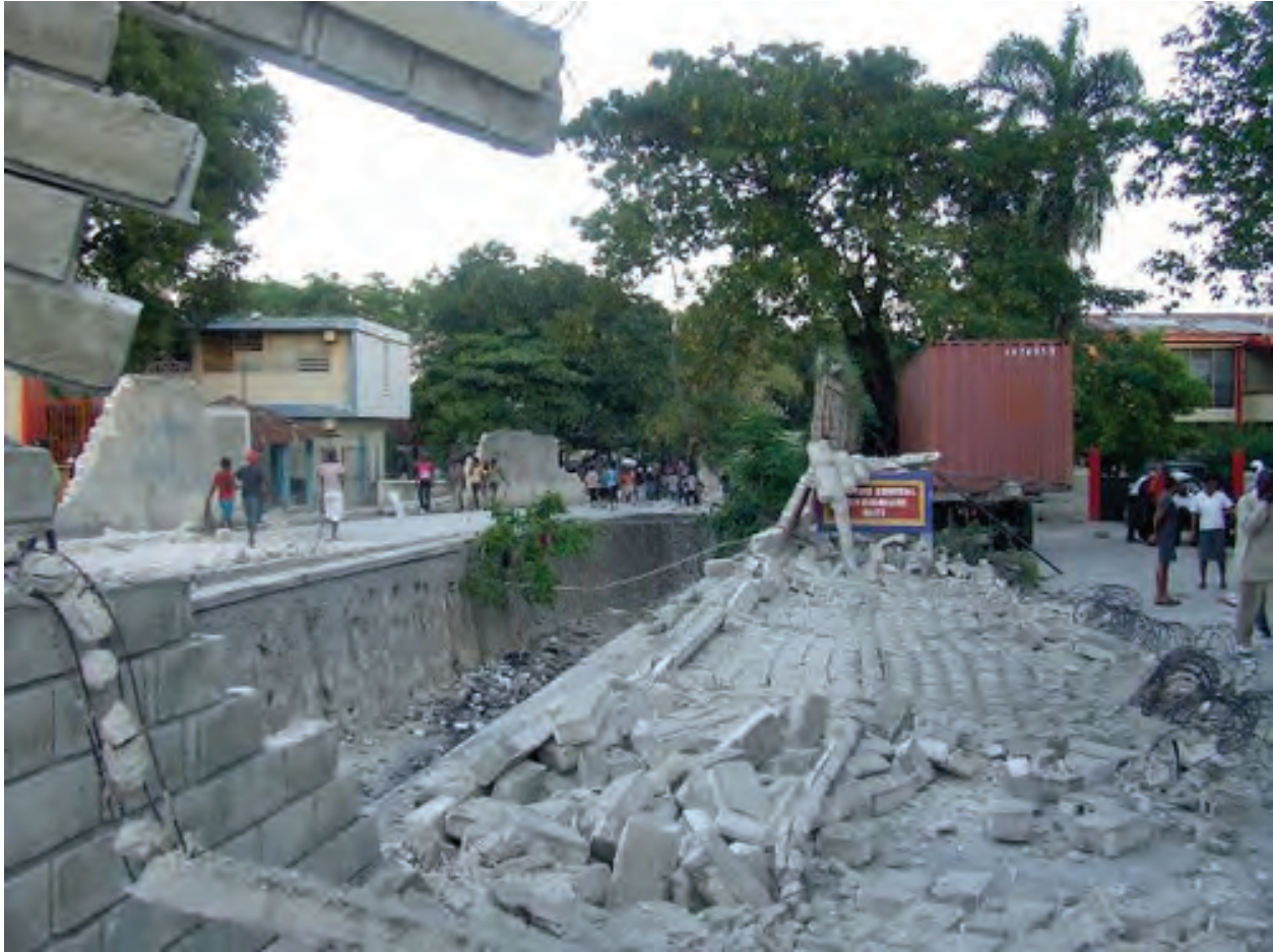
Figure 6.3.9.1-2 Freestanding masonry fences with inadequate reinforcement collapsed covering both sides of this street in Port-au-Prince in the 2010 magnitude-7 Haiti Earthquake (Photo courtesy of Yves Montoban). Many miles of such fencing collapsed in the 2010 Haiti Earthquake.
