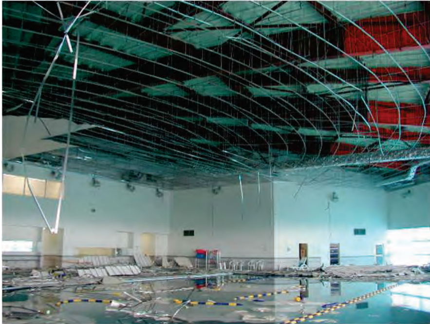
Figure 6.3.4.3-2a Complete collapse of a large suspended gypsum board ceiling over a swimming facility in Japan (Photo courtesy of Shojiro Motoyui, Tokyo Institute of Technology). This type of failure has been replicated on the E-defense shake table and occurs when the U-shaped clip holding the cross furring (M-bar) to the main runners (channel) opens into a V-shape and drops the furring grid. This type of failure is not common in the U.S.
