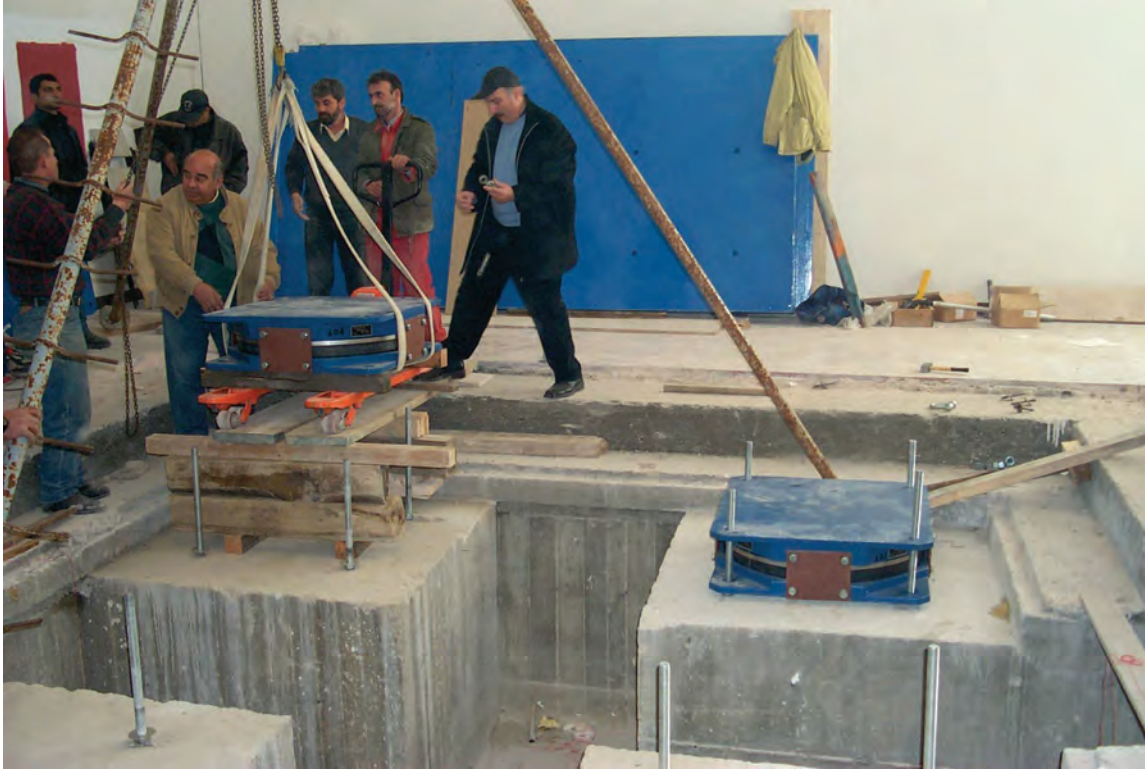
Figure 6.5.6.3-3b Installation of base isolation devices to support reinforced concrete slab for statue (Photo courtesy of University at Buffalo).
