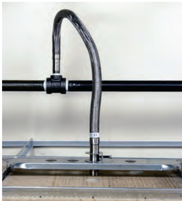
Figure 6.4.4.1-10 Flexible hose between sprinkler line and ceiling allowing the sprinkler head to move with the suspended ceiling without causing damage to the sprinkler system (Photo courtesy of Flexhead).
