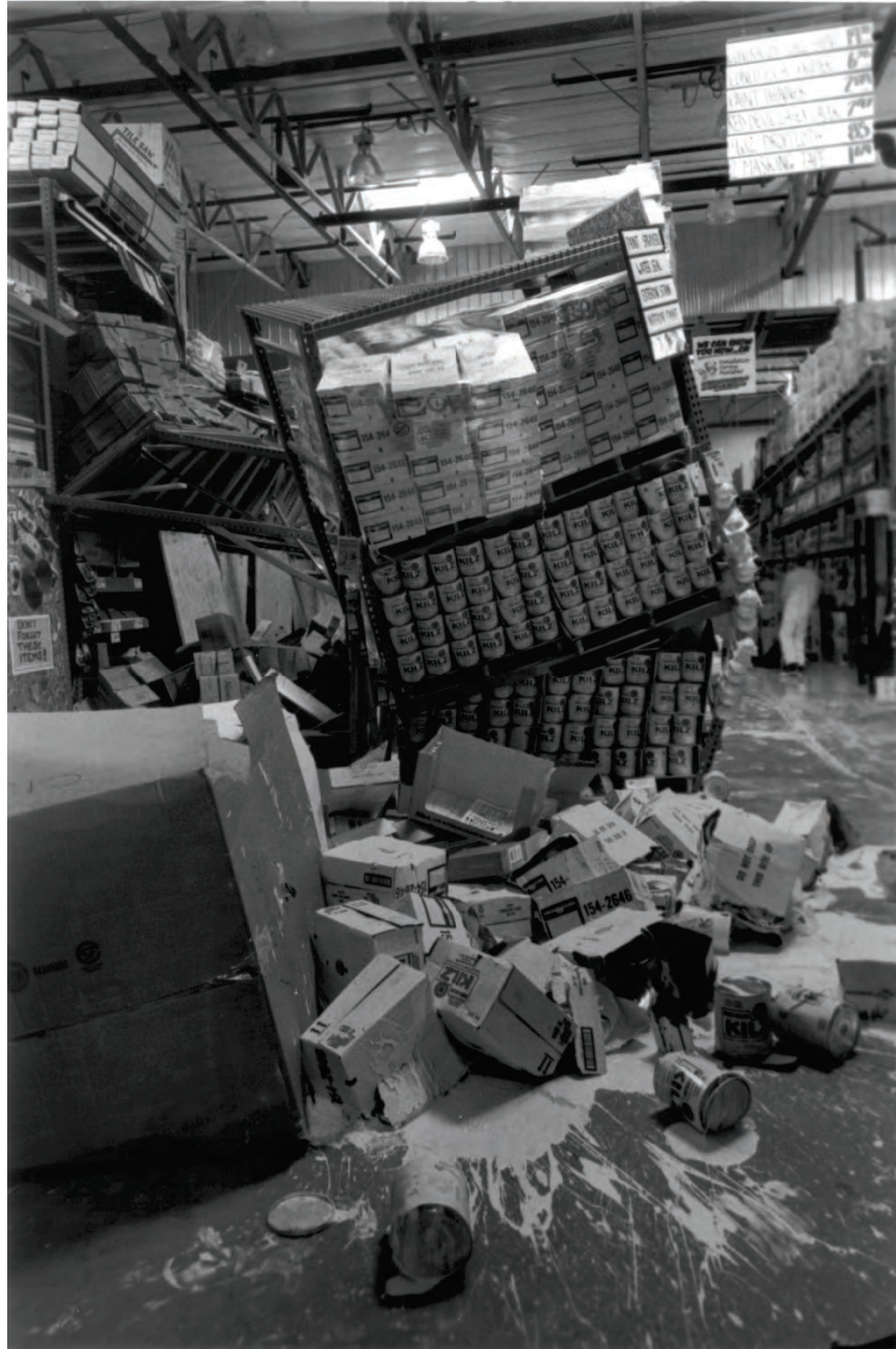
Figure 6.5.1.2-3 Rack collapse during the 1994 Northridge Earthquake. Note the minimal damage to shrink wrapped merchandise (FEMA 460, 2005).
