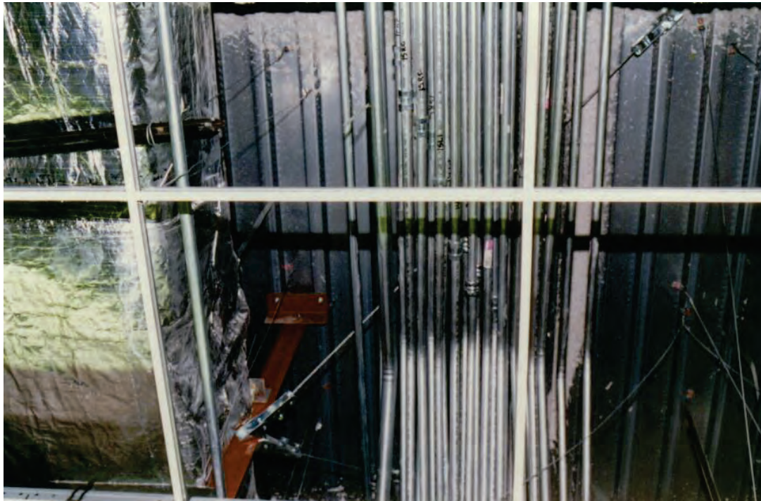
Figure 6.4.6.1-4 Rectangular duct supported by steel shapes with cable braces (Photo courtesy of Mason Industries).
