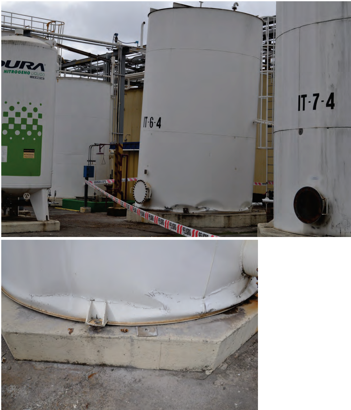
Figure 6.4.2.2-4 Anchored tank damaged at base when anchorage failed; tank slid and ruptured attached piping in 2010 magnitude-8.8 Chile Earthquake (Photo courtesy of Eduardo Fierro, BFP Engineers).
