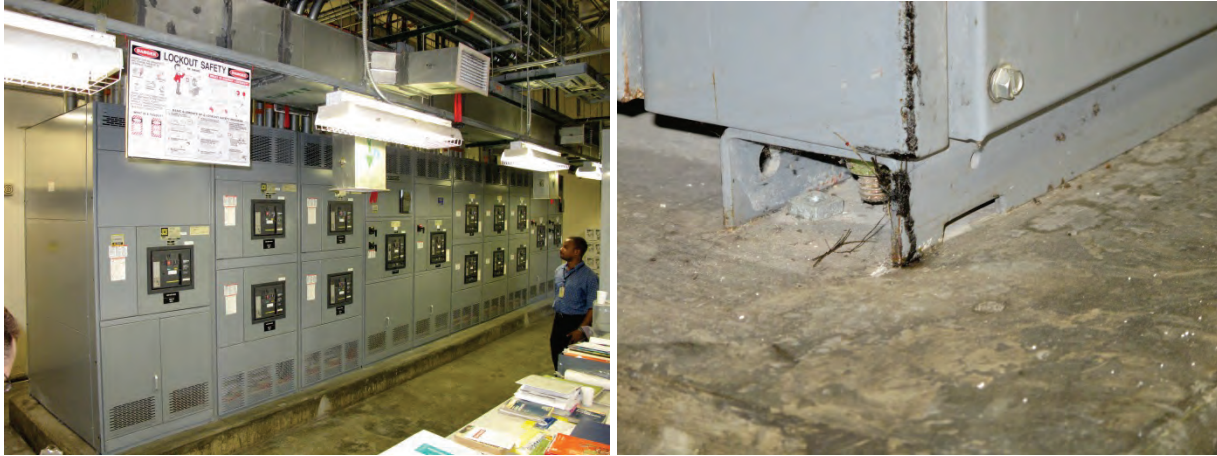
Figure 6.4.7.3-9 Incoming power switchgear for critical facility anchored through base undamaged by the 2010 Haiti M 7.0 Earthquake. Visual inspection of equipment base channels did not reveal any structural damage or equipment displacement on concrete equipment pad. Similar equipment located nearby which did not have a rigid seismic restraint with a continuous load path shifted on its pad (photos courtesy of Philip J. Caldwell).
