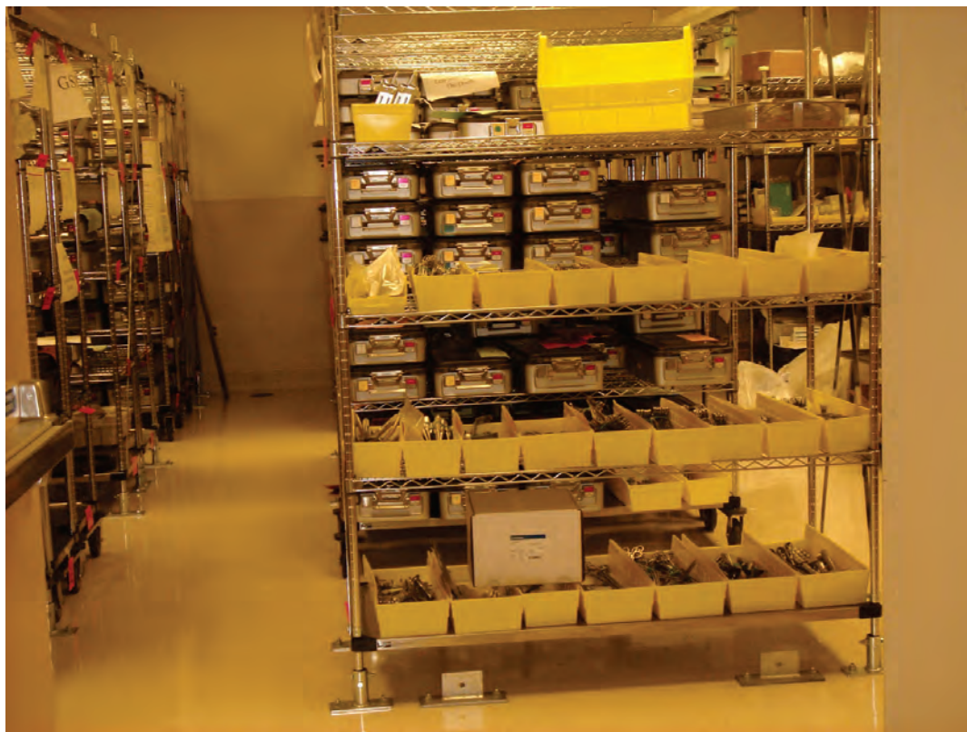
Figure 6.5.1.1-5 Fixed base shelving units anchored with optional seismic base plate offered by manufacturer (Photo courtesy of Maryann Phipps, Estructure).
