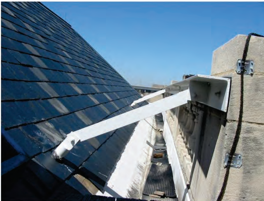
Figure 6.3.5.1-6 Close-up of parapet bracing (Photo courtesy of Degenkolb Engineers).
