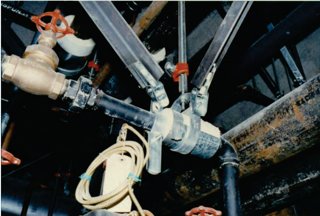
Figure 6.4.3.1-5 Pipe clamp supports with transverse and longitudinal angle braces; note pipe clamp for longitudinal brace in direct contact with pipe (Photo courtesy of Mason Industries).
