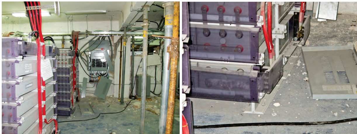
Figure 6.4.7.3-6 Battery room for central network cell phone carrier after 2010 M 7.0 Haiti Earthquake. Three-story building which contained the UPS (uninterruptable power supply) and battery room was newly constructed and suffered near collapse structural damage which required structural demolition and replacement. Note that high mass batteries with integral structural system was rigidly anchored and sustained no damage or loss of operation despite building structural system displacing enough to shear support columns. Cellular carrier representative advised that the central network support functionality was maintained during Earthquake (photos courtesy of Philip J. Caldwell).
