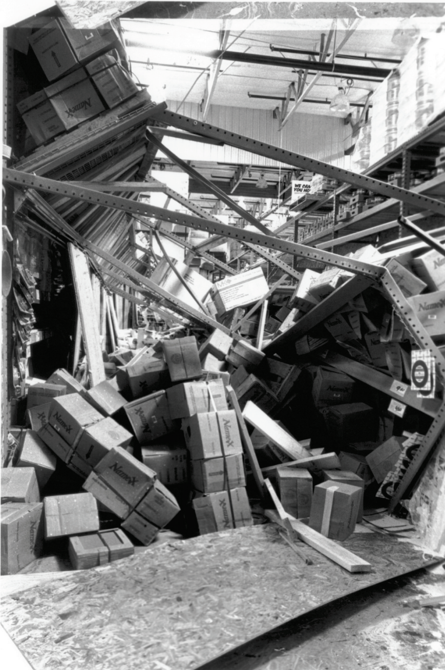
Figure 6.5.1.2-1 Damage to overloaded racks during the 1994 magnitude-6.7 Northridge Earthquake (FEMA 460, 2005).
