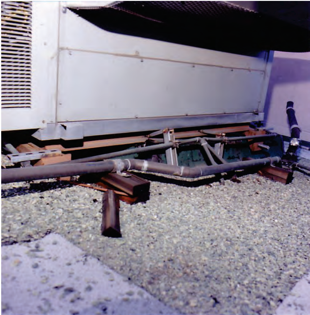
Figure 6.4.3.6-1 Damaged supports and piping on roof-mounted HVAC unit in the 1994 magnitude-6.7 Northridge Earthquake (Photo courtesy of Mason Industries). Both the roof-mounted wood sleepers and strut supports failed.
