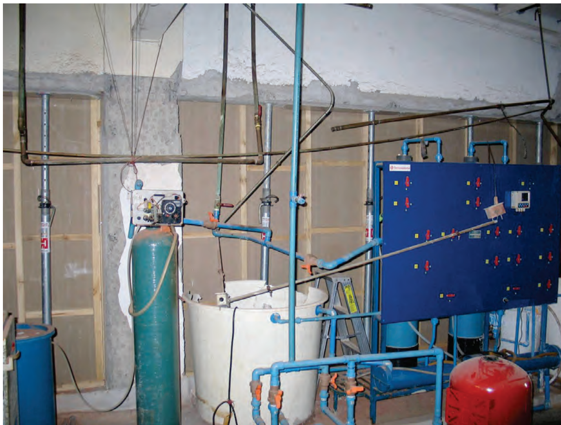
Figure 6.3.2.1-6 An infill masonry wall collapsed onto the distilled water equipment spilling two 150 gallon containers; water leaked past the perimeter edge of the floor slab into the operating room suite below resulting in the closure of 3 of 6 the operating rooms. Replacement gypsum board partition seen in photo. Hospital built in 2005 in Los Angeles, Chile. Damage from the 2010 Chile Earthquake (Photo courtesy of Bill Holmes, Rutherford & Chekene).
