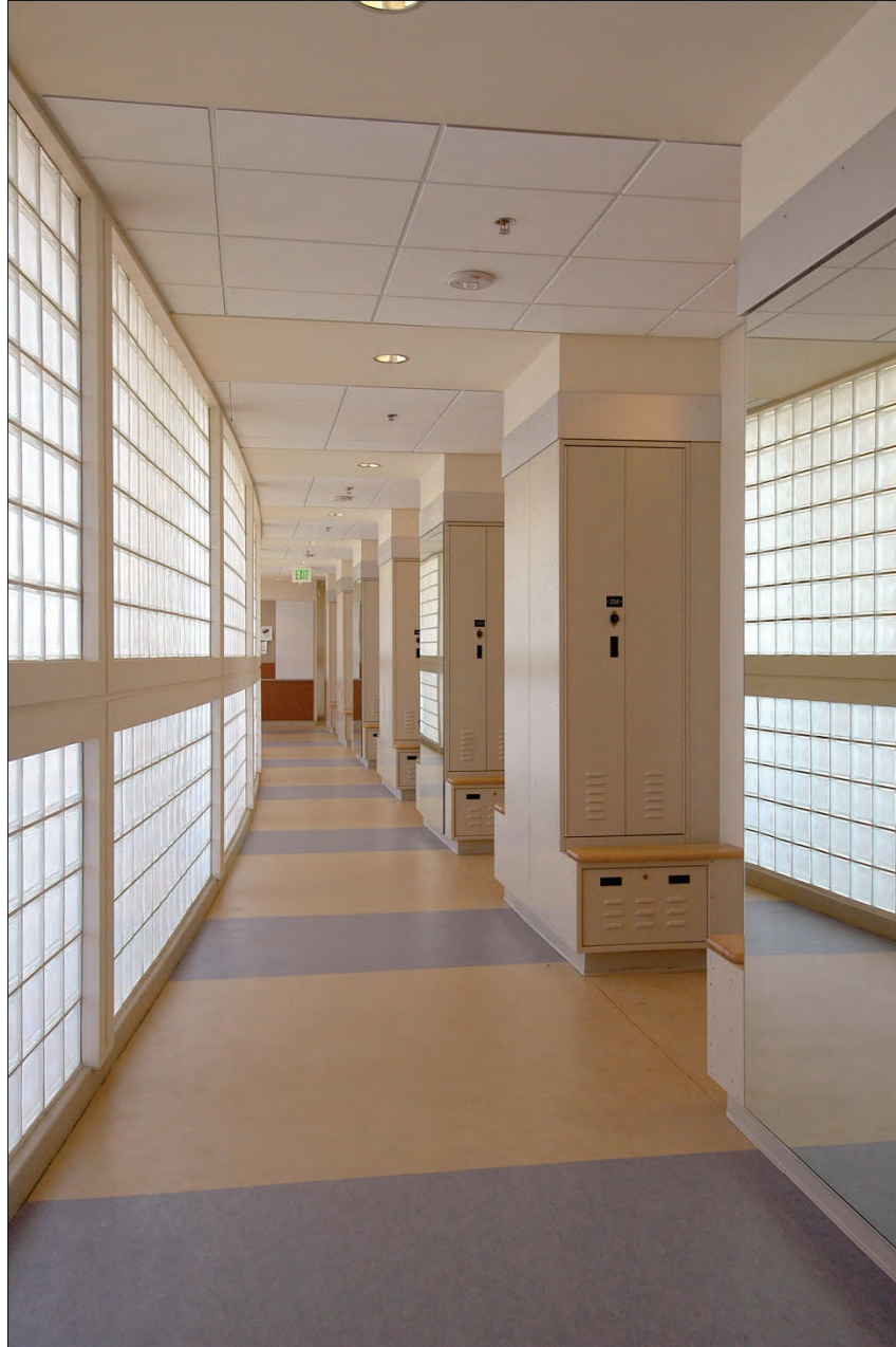
Figure 6.3.1.5-5 Glass block panels divided into numerous subpanels at the Chula Vista Police Headquarters, California (Photo courtesy of Pittsburgh Corning Corporation). In addition, the nonbearing glass block panel partition wall is isolated from seismic movement of the building structure.
