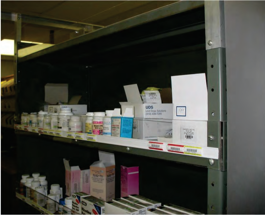
Figure 6.5.6.1-5 Plexiglass lip provides restraint for pharmaceuticals (Photo courtesy of Degenkolb Engineers).
