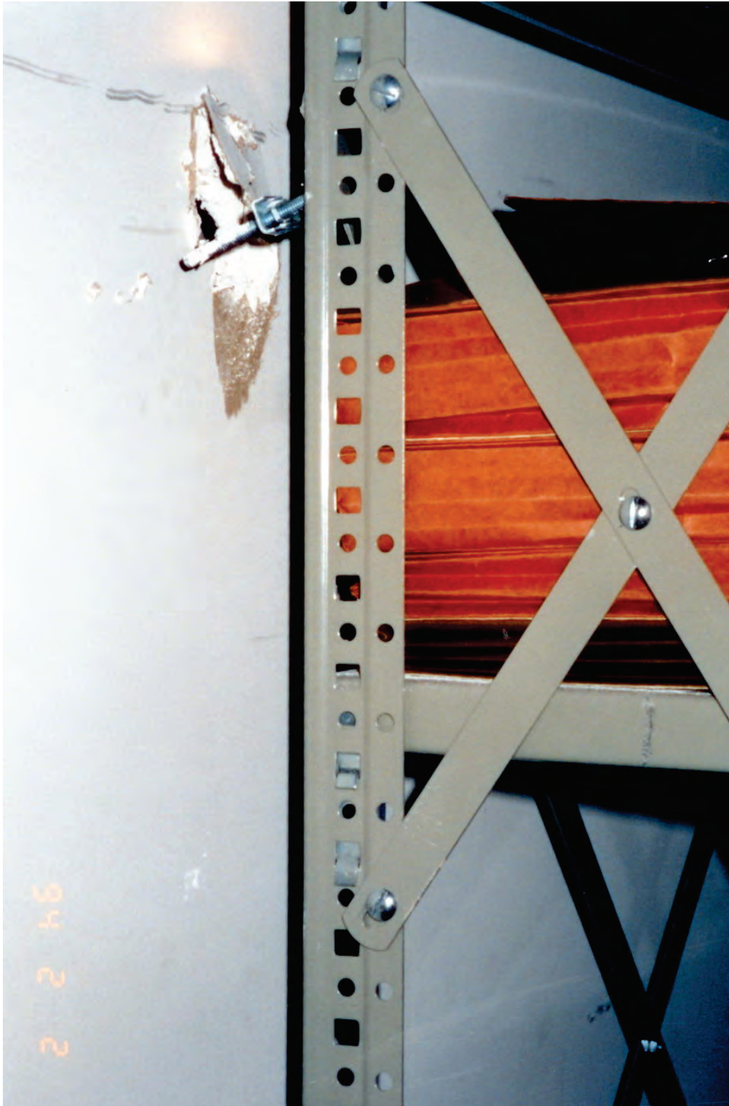
Figure 6.5.2.1-2 Failure of poorly anchored shelving; toggle bolt pulled out of gypsum board wall in the 1994 magnitude-6.7 Northridge Earthquake (Photo courtesy of Wiss, Janney, Elstner Associates).
