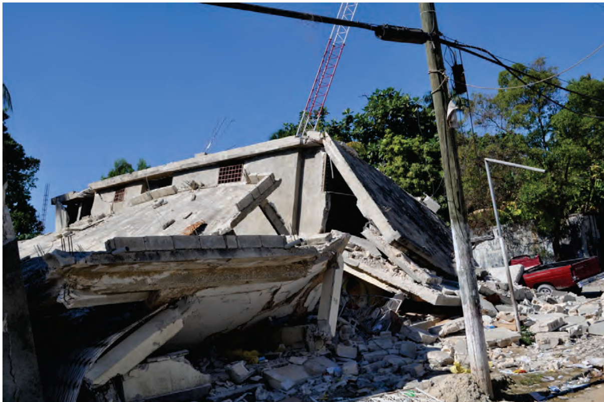
Figure 6.4.7.6-4 The antenna with guy wires remained upright atop a collapsed building in the 2010 Haiti Earthquake (Photo courtesy of Eduardo Fierro, BFP Engineers). Even though some of the guy wires went slack, the antenna did not fall into the street.
