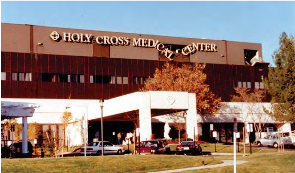
Figure 6.4.1.5-1 Damage to suspended HVAC, signs, and louvers was caused when suspended fans in the mechanical penthouse swung and impacted the louver panels. Holy Cross Medical Center in Sylmar, as a result of the 1994 magnitude-6.7 Northridge Earthquake (Photo courtesy of Robert Reitherman).
