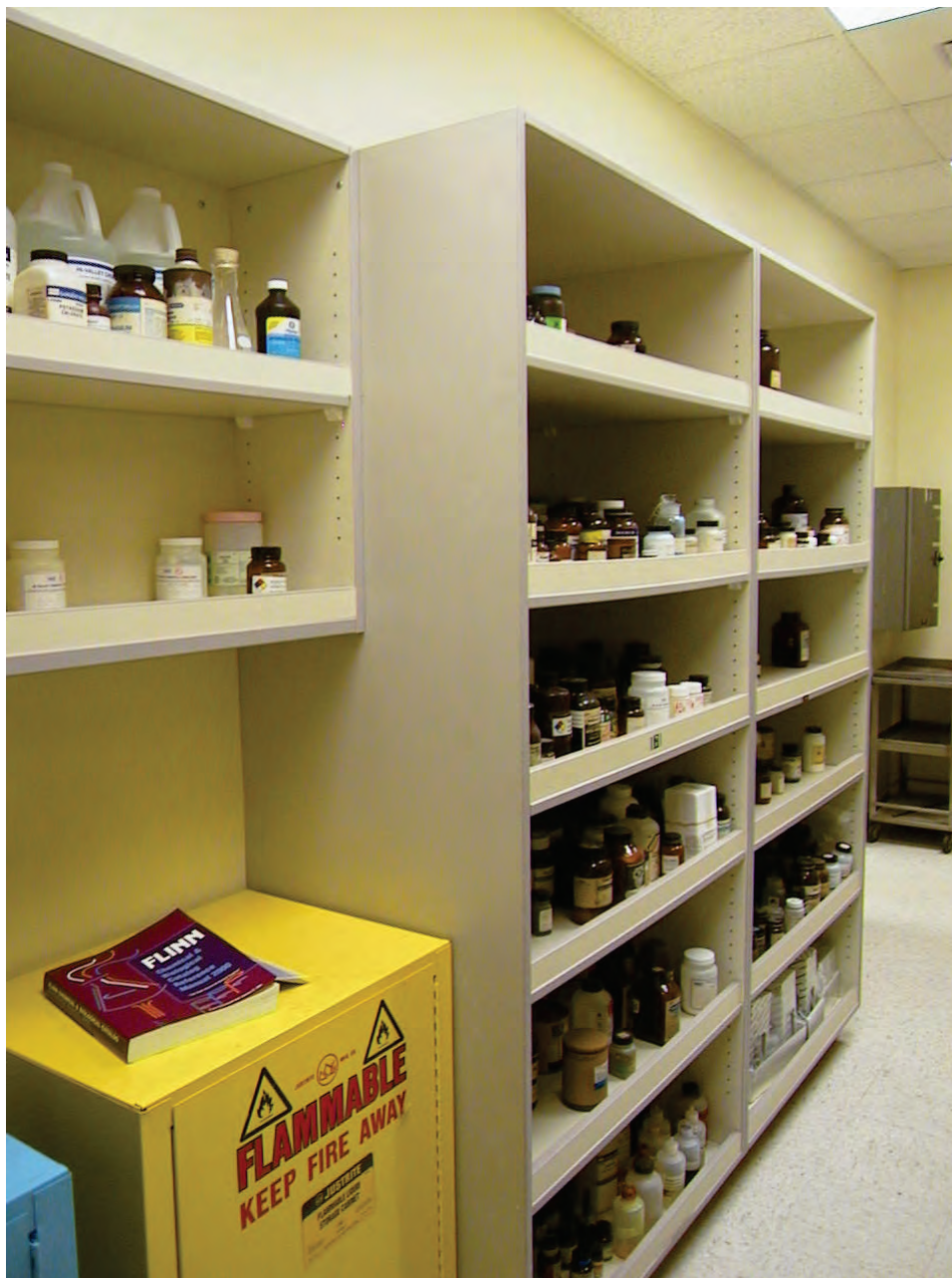
Figure 6.5.6.1-3 High school lab supplies protected on shelving with edge restraints (Photo courtesy of EQE for the Salt Lake City School District).
