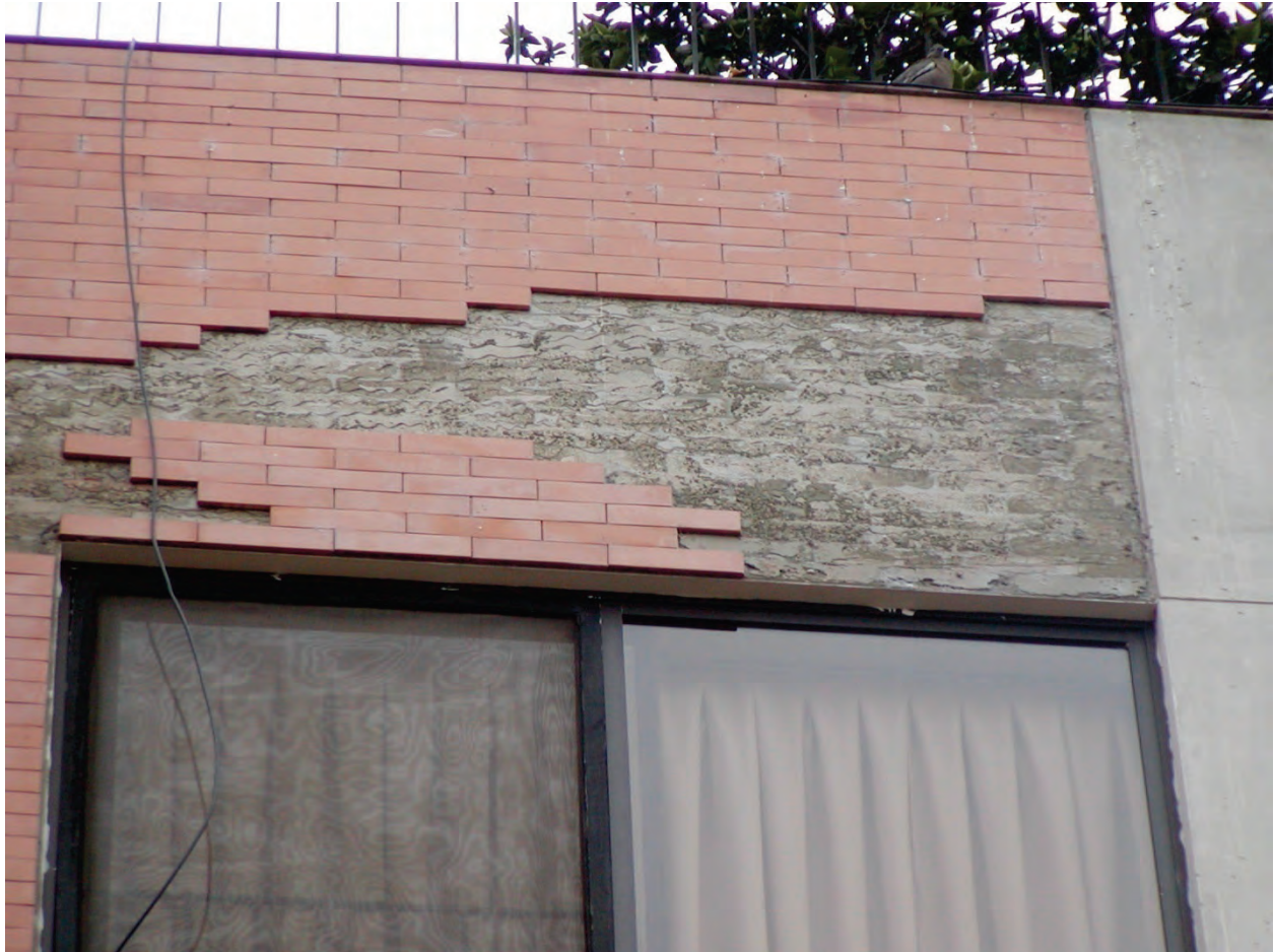
Figure 6.3.1.1-2 Close-up of failed adhered veneer. (Photo courtesy of Eduardo Fierro, BFP Engineers).
