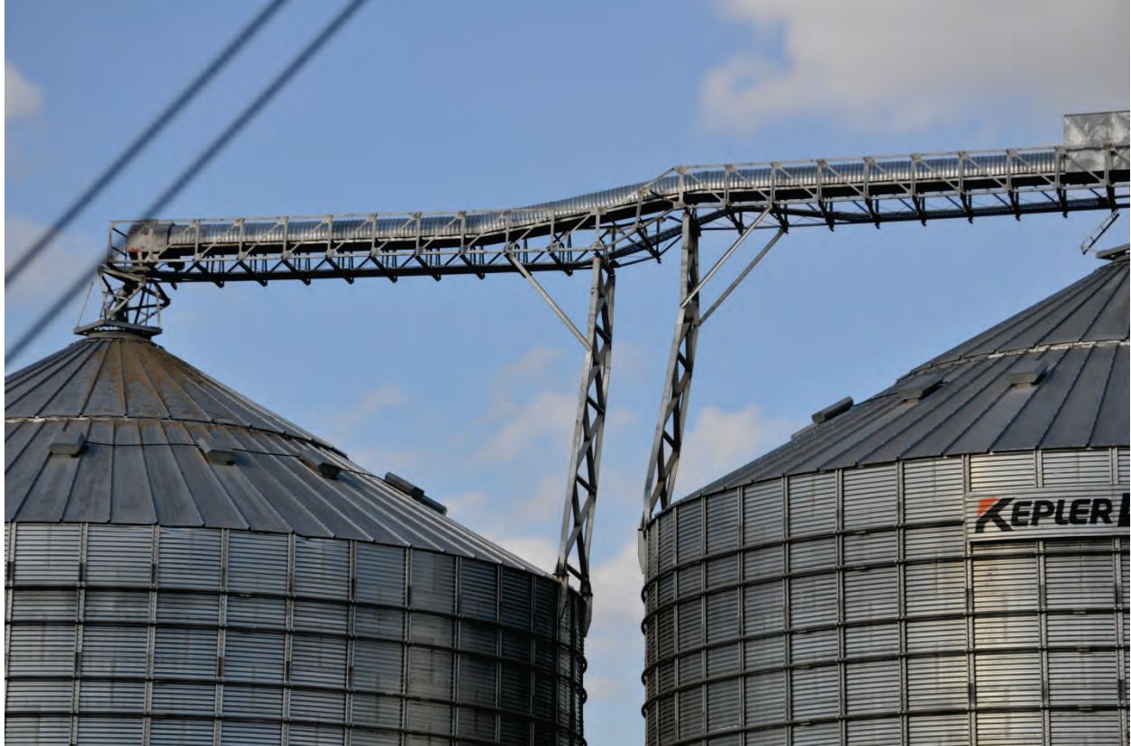
Figure 6.4.11.1-2 Damage to industrial conveyor used to feed grain silos in the 2010 Chile Earthquake (Photo courtesy of Eduardo Fierro, BFP Engineers).
