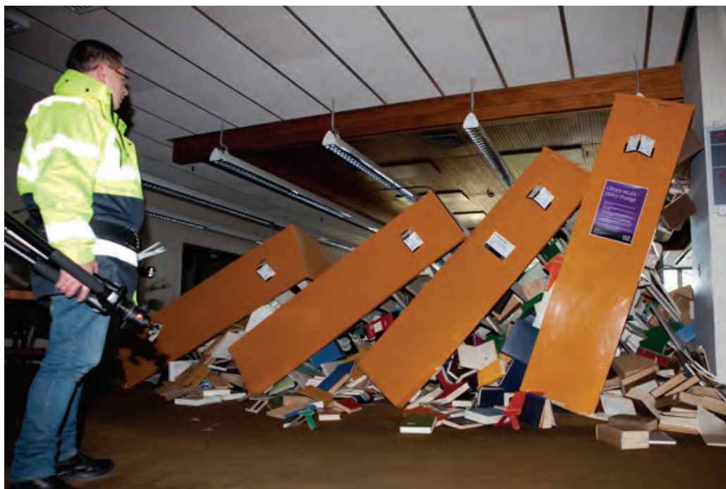
Figure 6.5.2.2-1 Photo showing collapsed library shelving in the 2010 magnitude-7.1 Canterbury New Zealand Earthquake (Photo courtesy of University of Canterbury).
