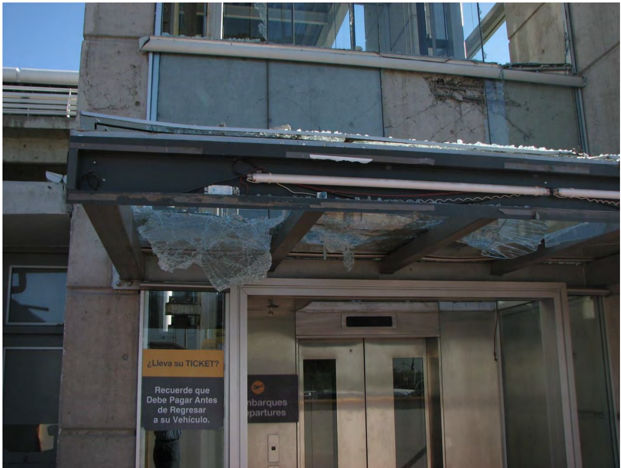
Figure 6.4.10.2-10 Glazing failures caused additional hazards at Santiago airport elevator in the 2010 Chile Earthquake (Photo courtesy of Antonio Iruretagoyena, Rubén Borsochek & Associates).
