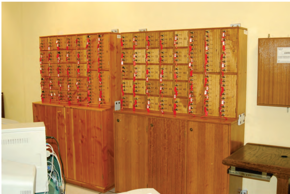
Figure 6.5.5.3-4 Anchored wood key cabinets in industrial plant control room; note top and bottom units anchored together and both anchored to wall (Photo courtesy of Eduardo Fierro, BFP Engineers).
