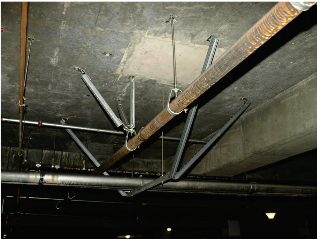
Figure 6.4.3.1-7 Transverse bracing with J-hanger and strut at the restraining bolt. Note that longitudinal brace shown is ineffective because the J-hanger can slip along the length of the pipe; a pipe clamp or equivalent is required for a longitudinal brace (Photo courtesy of Cynthia Perry, BFP Engineers).
