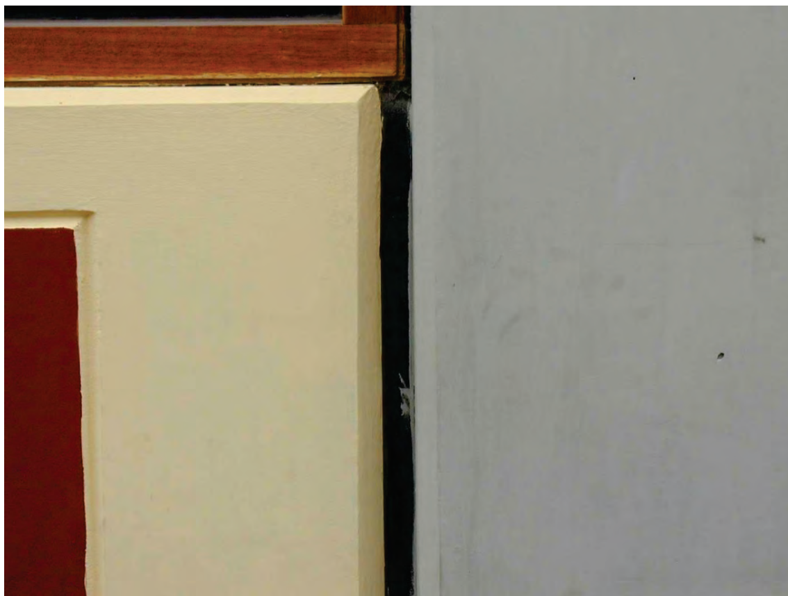
Figure 6.3.2.1-7 Detail of isolation joint to prevent creation of “captive column” condition (Photo courtesy of Eduardo Fierro, BFP Engineers).
