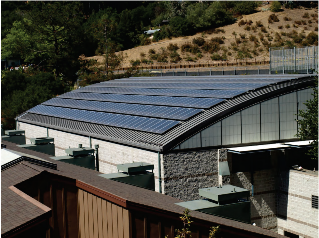
Figure 6.4.7.5-4 Flush mount photovoltaic system on barrel shaped roof of gymnasium at Head-Royce School, Oakland, California (Photo courtesy of Cynthia Perry, BFP Engineers).
