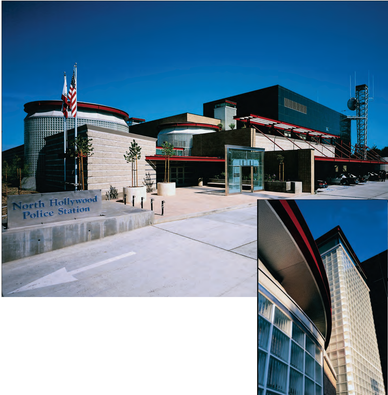
Figure 6.3.1.5-4 Use of glass block panels for select exterior and interior walls at the North Hollywood Police Station in California, utilizing standard details provided by Pittsburgh Corning Glass (Photo courtesy of Pittsburgh Corning Corporation).
