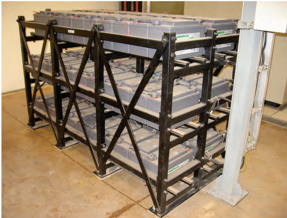
Figure 6.4.7.4-4 Battery rack that performed well in the 2010 magnitude-8.8 Chile Earthquake (Photo courtesy of Rodrigo Retamales, Rubén Boroschek & Associates).
