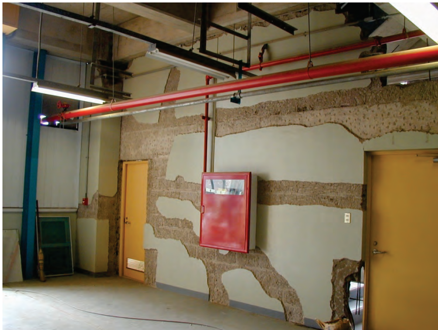
Figure 6.3.2.1-2 Damage to reinforced concrete masonry partition used to support fire protection cabinet and piping in the 2001 Peru Earthquake; loose stucco and masonry were removed prior to photo (Photo courtesy of Eduardo Fierro, BFP Engineers).
