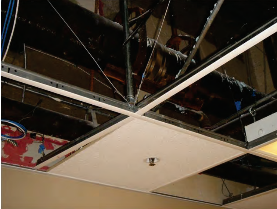
Figure 6.3.4.1-6 Compression struts and diagonal splayed wires are used to limit the movement of suspended acoustic tile ceilings. Per ASTM E580, this type of bracing assembly is required for ceiling areas larger than 1000 sq. ft. in Seismic Design Category D,E, and F (Photo courtesy of Maryann Phipps, Estructure).
