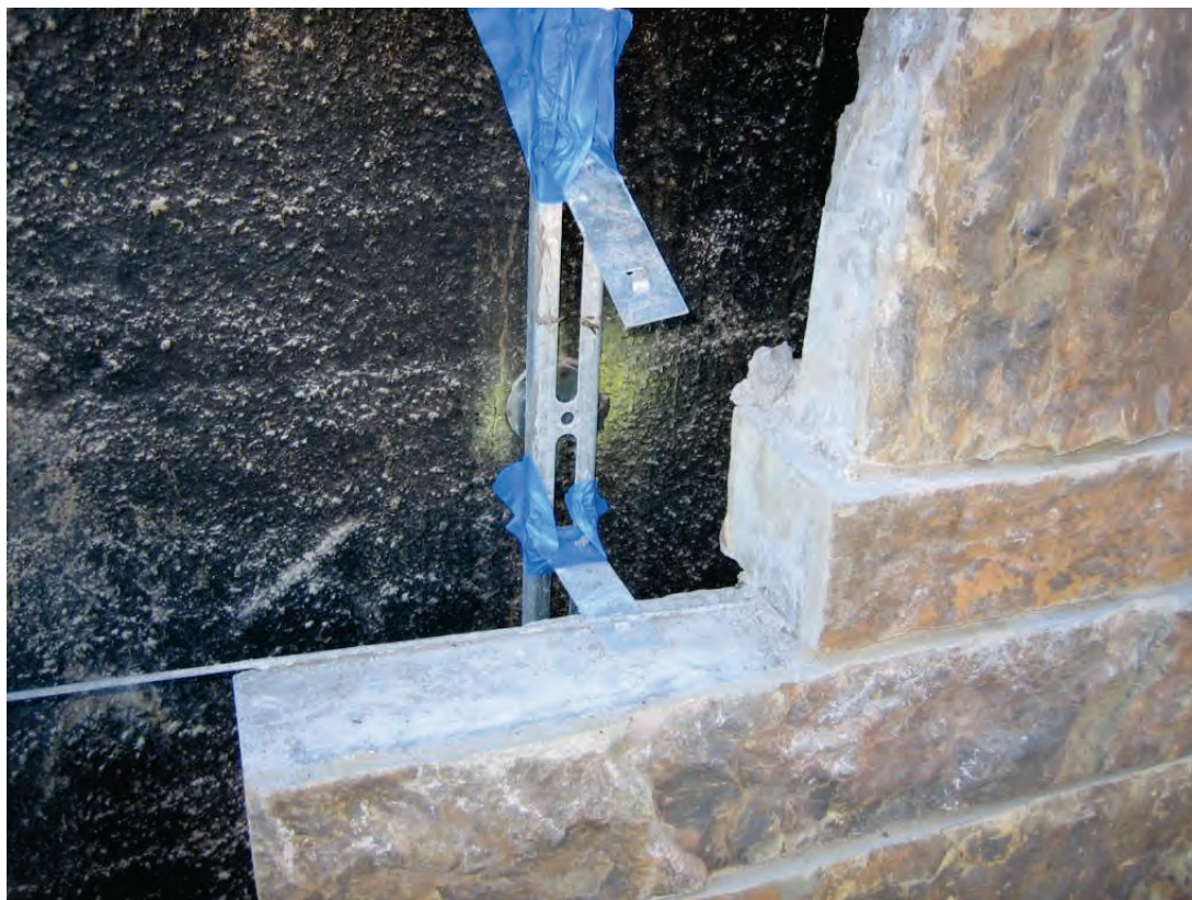
Figure 6.3.1.2-4 Installation of stone veneer showing anchorage to steel dovetail clips which are fastened to steel studs bolted to the grouted reinforced masonry wall behind (Photo courtesy of Simpson Gumpertz and Heger).
