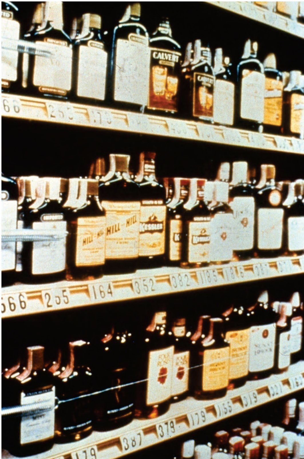
Figure 6.5.6.1-4 Shelf restraint example; shock cord made of wire and springs used to restrain liquor bottles (Photo courtesy of Robert Reitherman).
