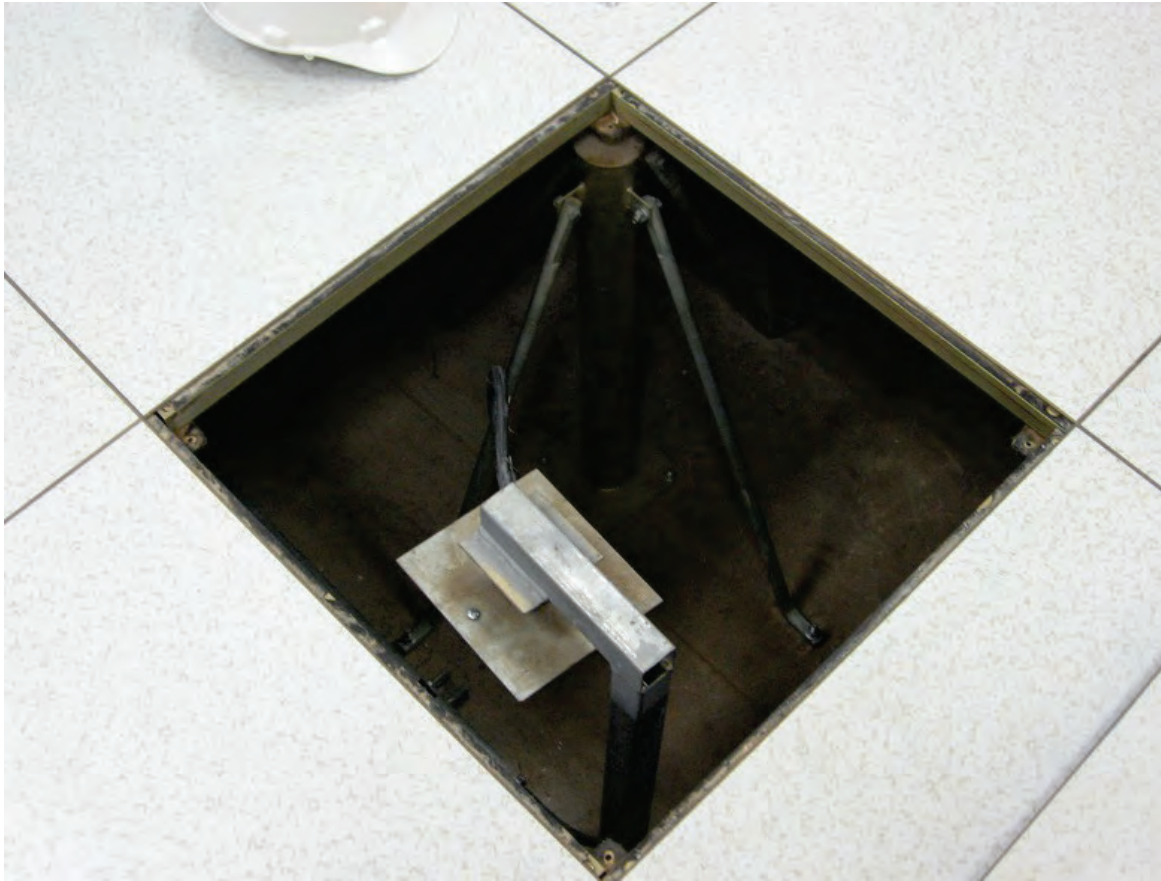
Figure 6.5.3.1-3 Undamaged access floor with braced pedestals in the 2010 Chile Earthquake (Photo courtesy of Rodrigo Retamales, Rubén Boroschek & Associates).
