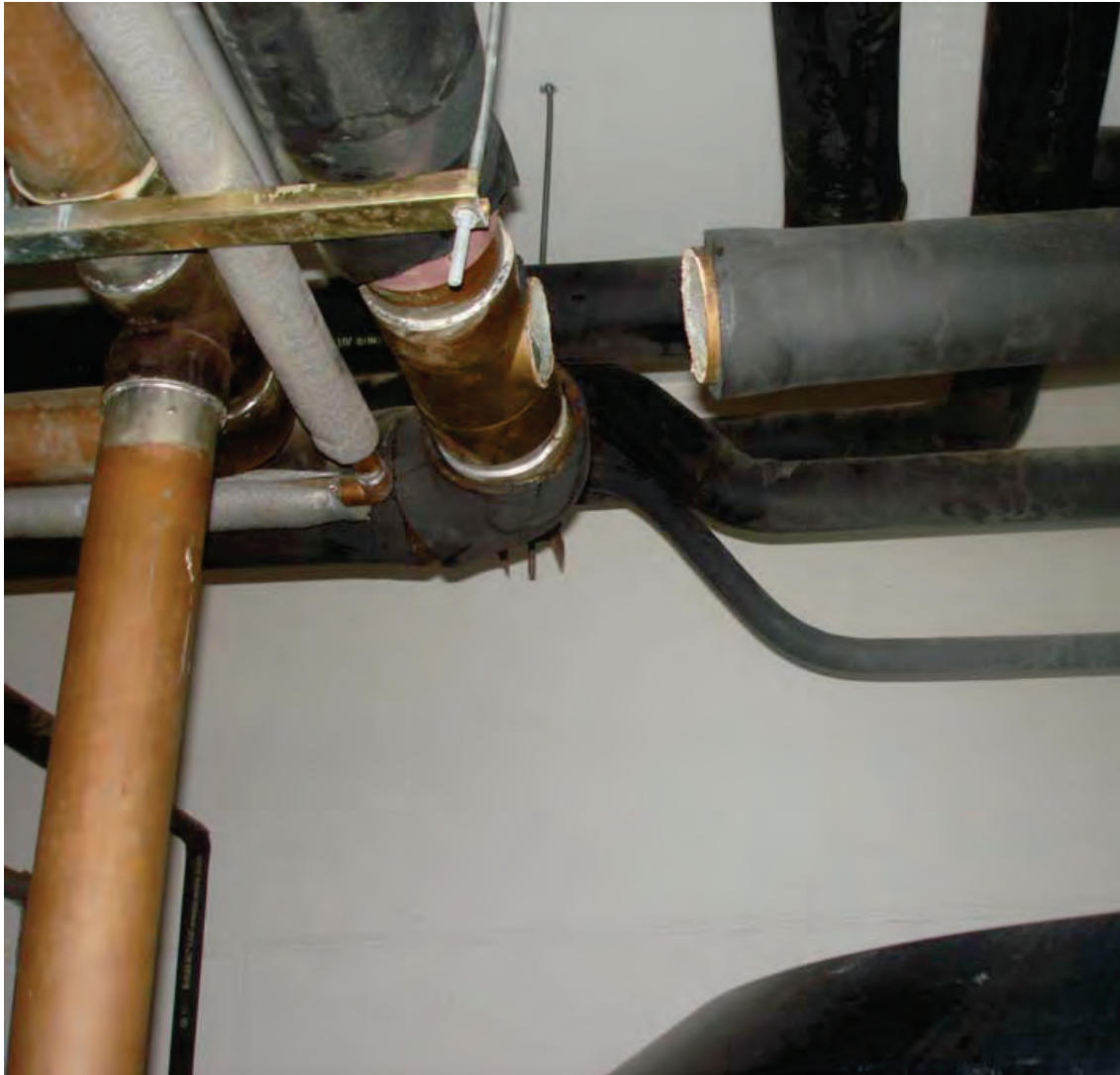
Figure 6.4.5.2-2 Broken copper piping for hot water supply in residential building in the 2010 Chile Earthquake. Trapeze shown not laterally braced but hangers appear to be less than 12" in length and may not have required lateral restraints per ASCE 7-10 (Photo courtesy of Gokhan Pekcan).
