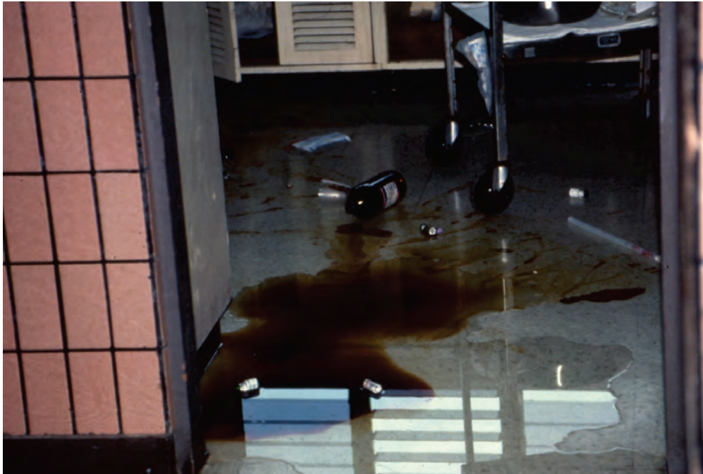
Figure 6.5.4.1-3 Spilled fluids in a hospital in the Costa Rica Earthquake (Photo courtesy of Degenkolb Engineers).
