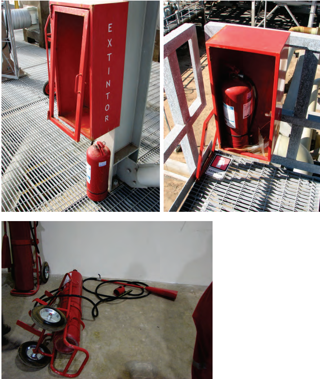
Figure 6.5.6.4-1 Fire extinguishers damaged during the 2010 magnitude-8.8 Chile Earthquake at an industrial facility (Photos courtesy of Antonio Iruretagoyena, Rubén Boroschek & Associates).
