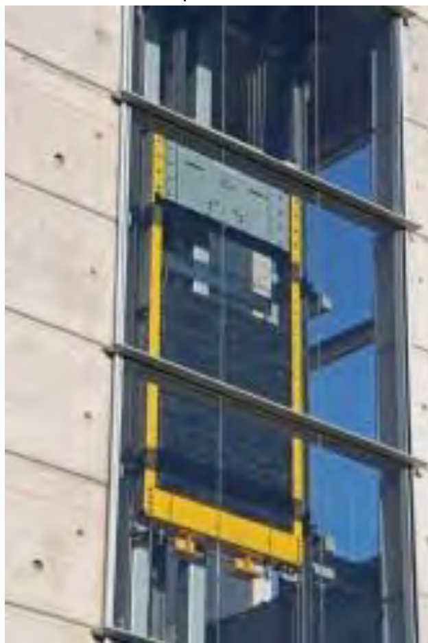
Figure 6.4.10.2-1 Examples of an elevator counterweight (Photo courtesy of Eduardo Miranda, Stanford University).
