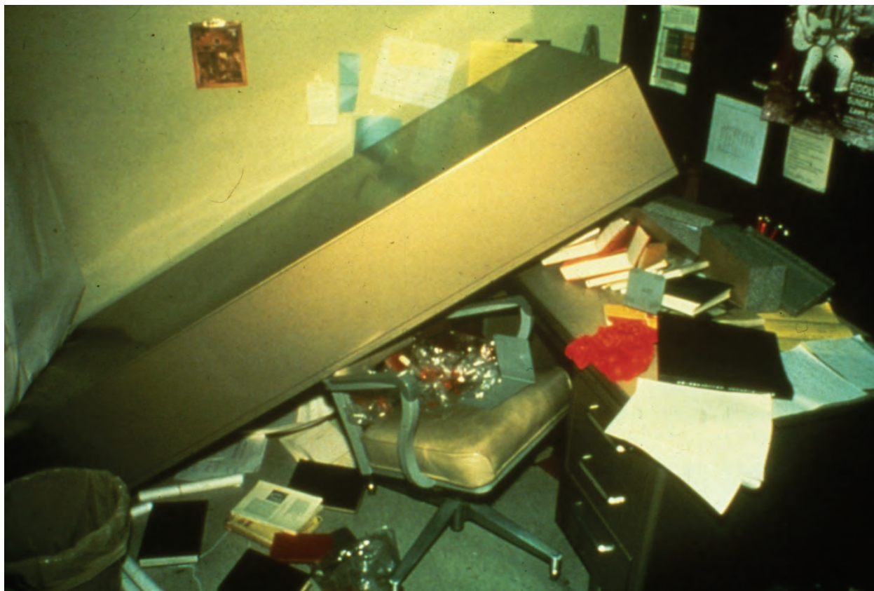
Figure 6.5.2.1-3 Bookcase overturned onto desk in the 1971 magnitude-6.6 San Fernando Earthquake (Photo courtesy of Degenkolb Engineers).
