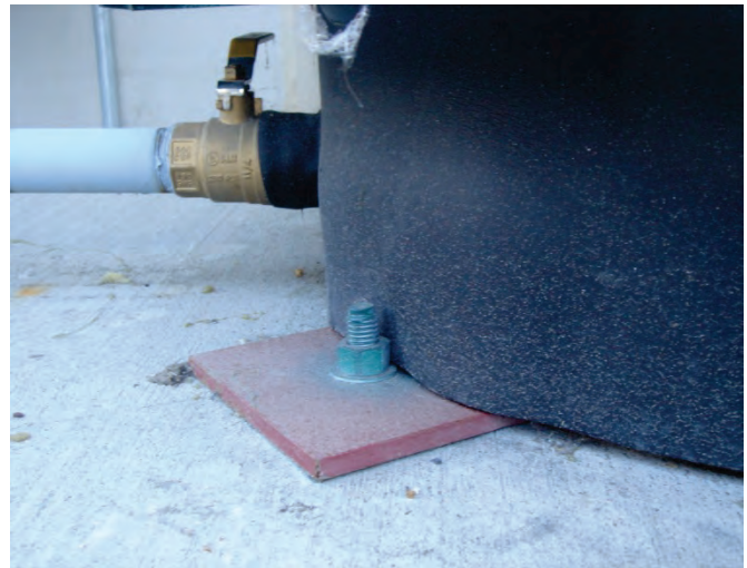
Figure 6.4.2.2-7 Examples of rigid base anchorage for small circular tanks (Photos courtesy of Maryann Phipps, Estructure).
