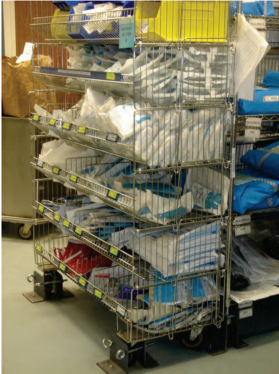
Figure 6.5.1.1-6 Mobile cart restrained at base with removable angles and eyebolts. Back-to-back units are interconnected (Photo courtesy of Maryann Phipps, Estructure).
