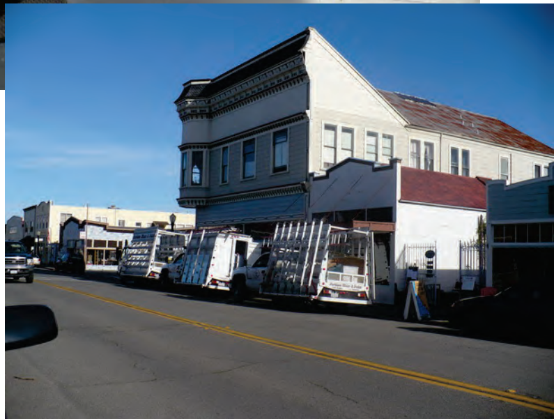
Figure 6.3.1.4-2 Scenes in Ferndale, California following the 2010 magnitude-6.5 Eureka Earthquake. 50% of the glazing on Main Street was cracked (Photos courtesy of Bret Lizundia, Rutherford & Chekene).
