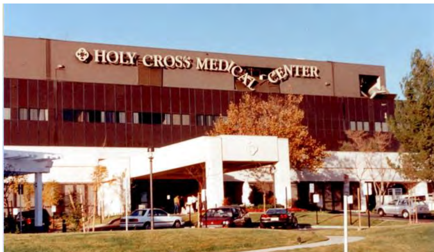
Figure 2.4.3-2 HVAC damage at Holy Cross Medical Center in Sylmar in the 1994 Northridge Earthquake. Damage to signage and louvers was caused when suspended fans in the mechanical penthouse swung and impacted the louver panels. HVAC service outage caused the temporary evacuation of patients (FEMA 74, 1994).
