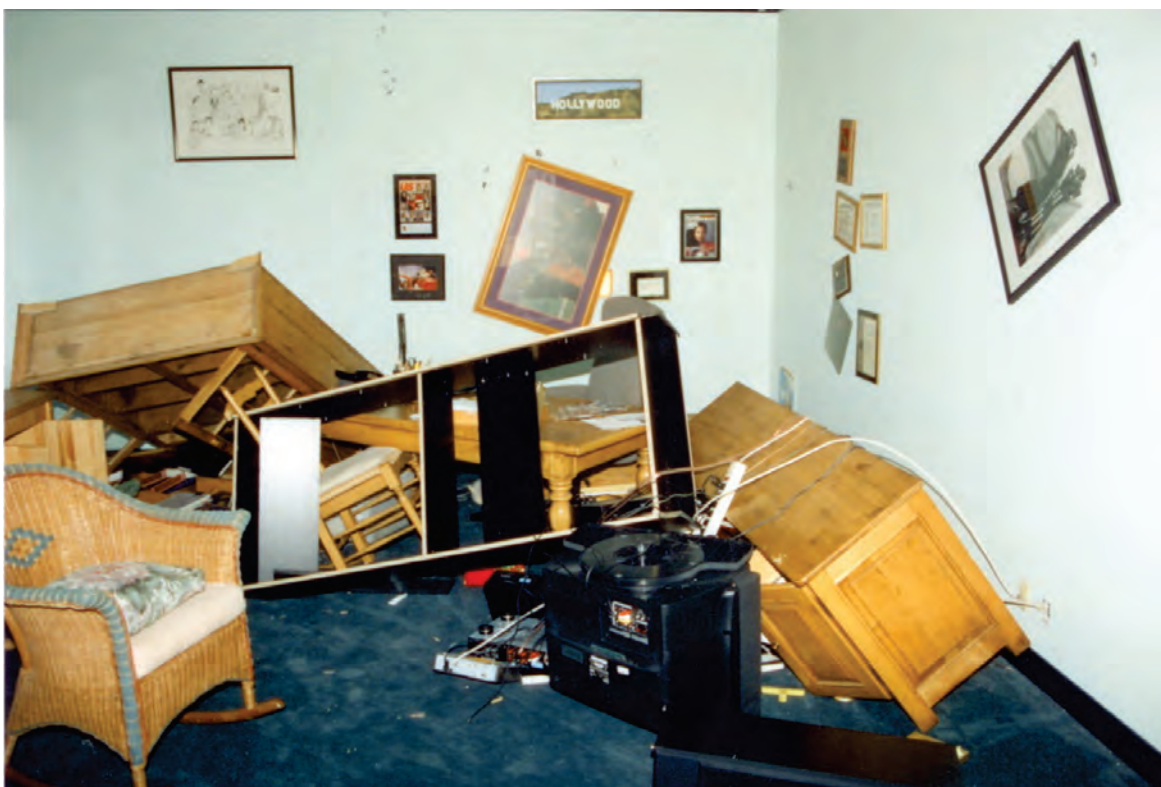
Figure 6.5.5.3-1 Residential damage in the 1994 magnitude-6.7 Northridge Earthquake (Photo courtesy of Wiss, Janney, Elstner Associates).
