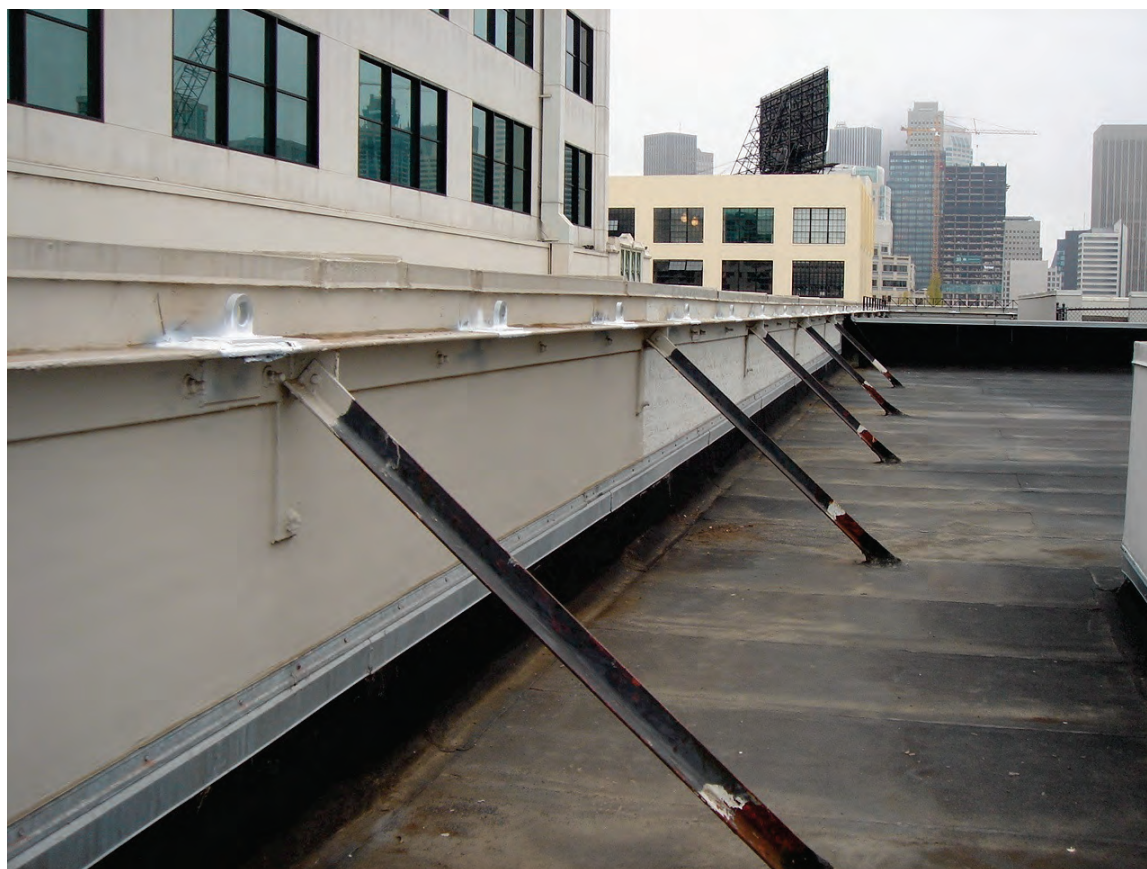
Figure 6.3.5.1-4 Bracing of URM parapet (Photo courtesy of Maryann Phipps, Estructure).
