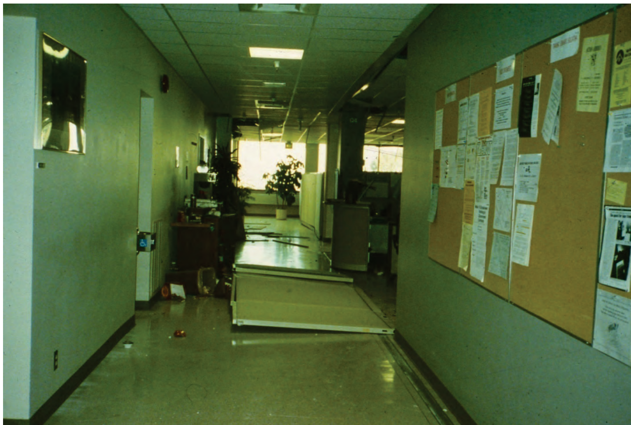
Figure 6.5.5.2-2 Damage to unbraced demountable partition in Silicon Valley office building in the 1989 magnitude-6.9 Loma Prieta Earthquake (Photo courtesy of Maryann Phipps, Estructure).
