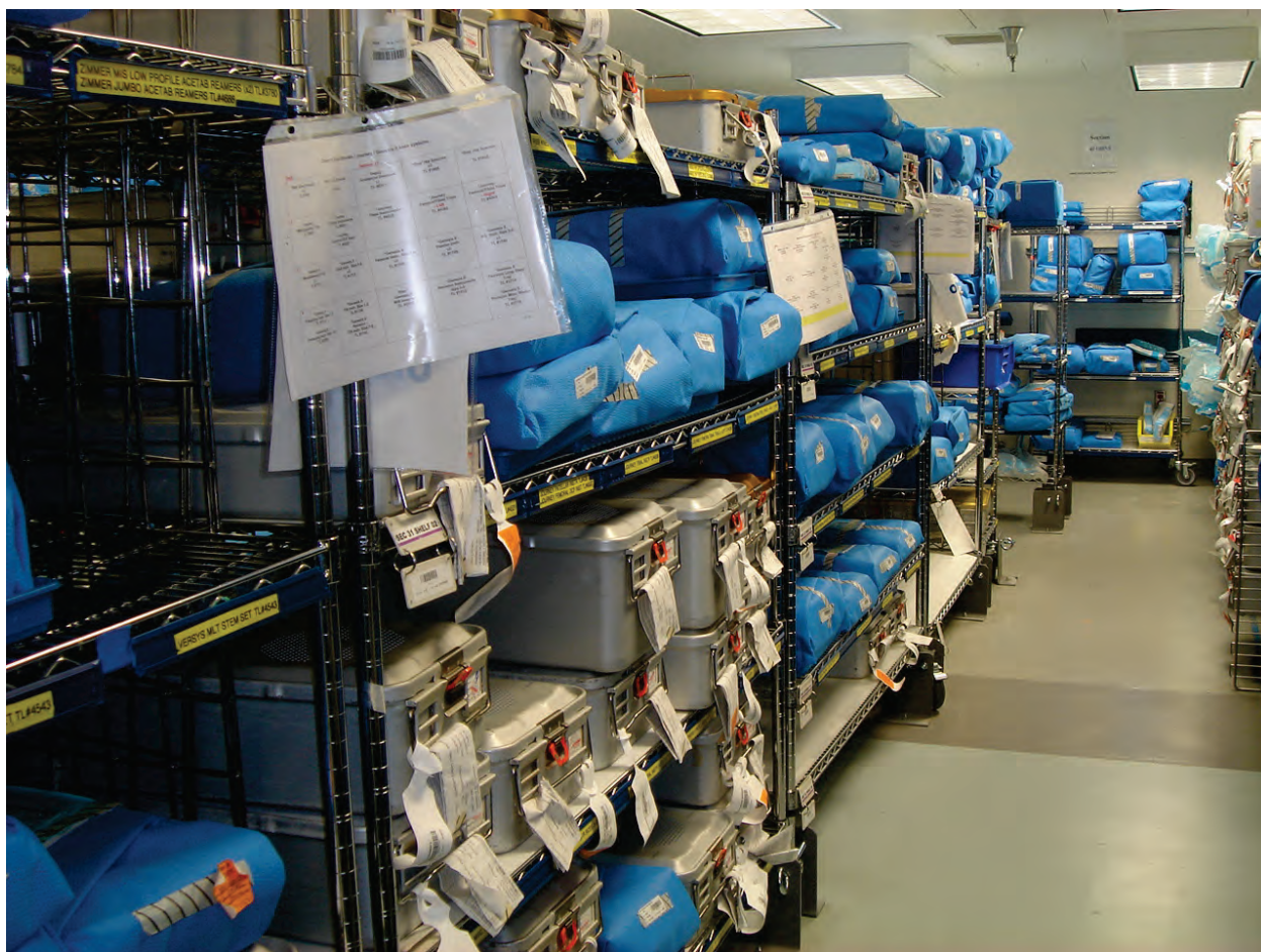
Figure 6.5.1.1-3 Mobile carts restrained at base with clip angles anchored to the floor and removable eyebolts attached from each cart to the angles (Photo courtesy of Maryann Phipps, Estructure).
