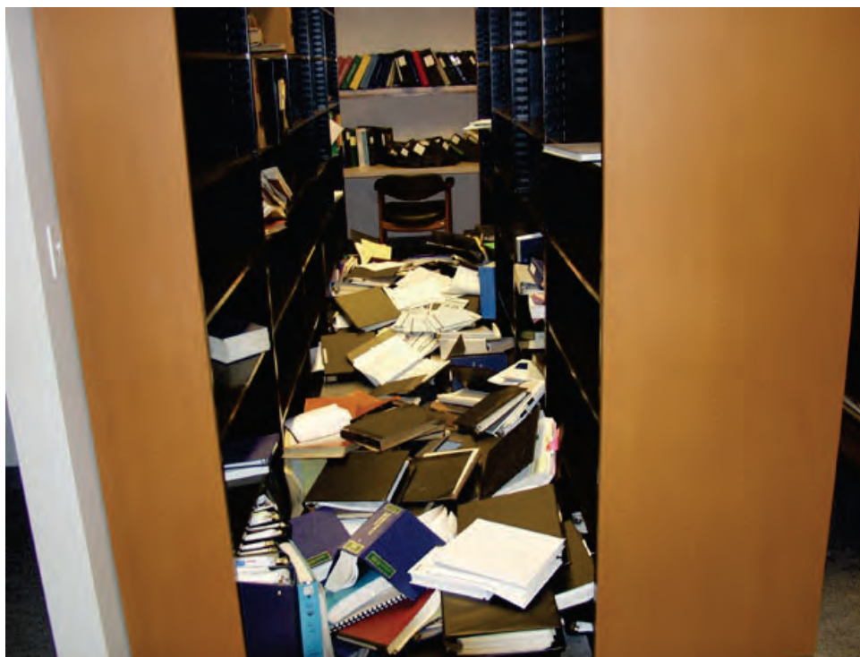
Figure 6.5.2.2-5 These shelving units remained in place but all of the contents spilled in the 2010 magnitude-6.5 Eureka, California Earthquake (Photo courtesy of Steve Mahin, PEER).
