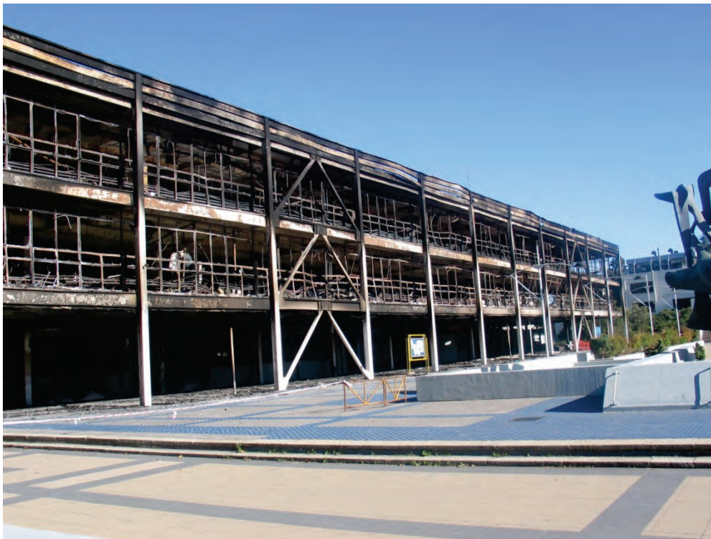
Figure 6.5.4.1-4 Fire destroyed the chemistry building containing the entire chemistry department at the University of Concepción in the 2010 magnitude-8.8 Chile Earthquake; fire exacerbated by the presence of hazardous chemicals (Photo courtesy of Bill Holmes, Rutherford & Chekene).
