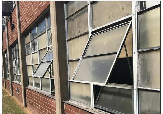
Open windows at a Maryland school without air conditioning in most areas of the building. The school district must close school if the building temperature rises above a safe level for students and staff.
