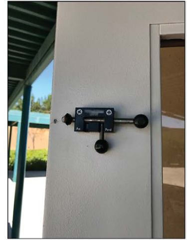
Door hardware that allows the door to be locked quickly in an emergency at a school in California.
