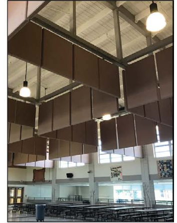
Acoustical panels dampen cafeteria noise levels in a Maryland school.
