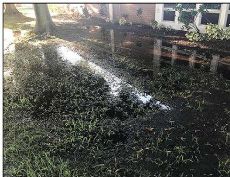
Standing water after a storm outside a school in Florida. School personnel work to clear drains and place sandbags in an attempt to mitigate water intrusion and flooding.
