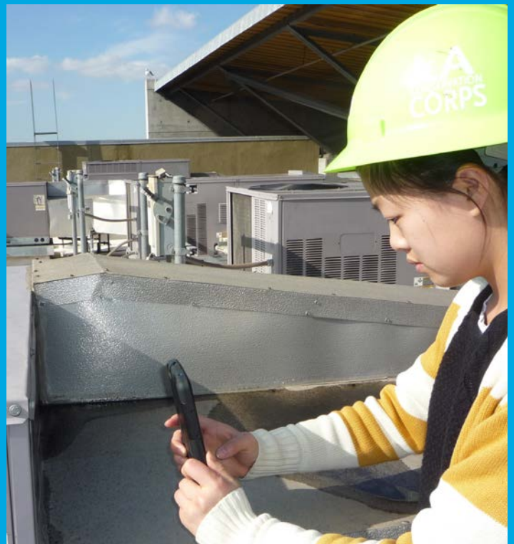
After learning about safety and security, Student Energy Auditor Training program students at LAUSD spend time inspecting HVAC systems and learning how to review and collect data. Photo by LAUSD
