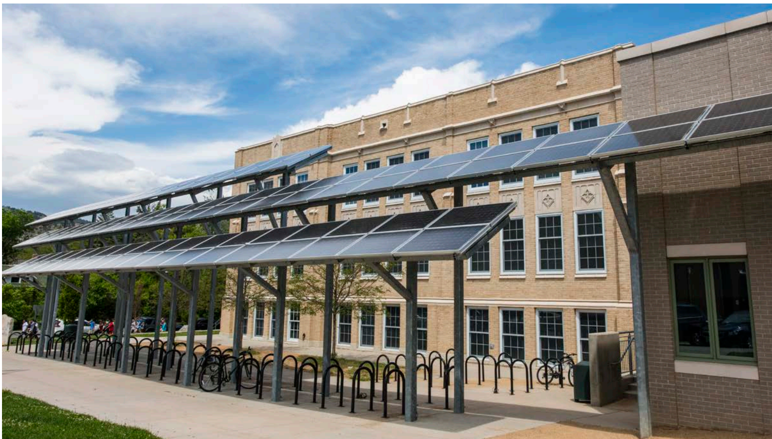
Casey Middle School, a LEED Platinum facility in Boulder, Colorado, features a 27-kW solar bike port. Photo by Dennis Schroeder, NREL 45244
