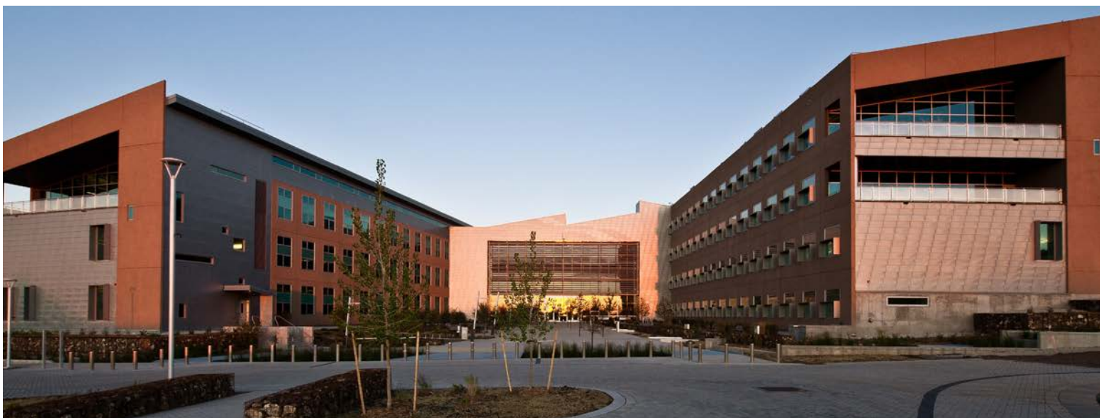
The National Renewable Energy Laboratory's Research Support Facility is a zero energy office building that cost the same to build as a conventional building. Photo by Dennis Schroeder, NREL 45244
