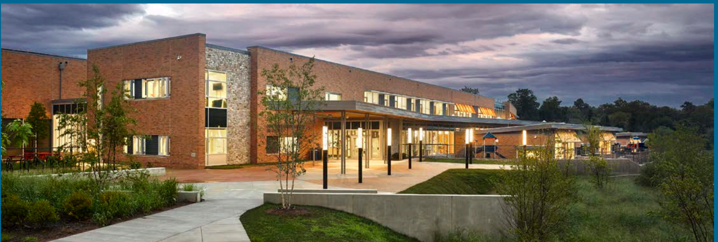
The success of Discovery Elementary School, a zero energy school in Arlington, Virginia, has been the impetus for other ZE schools in the area. Photo from VMDO Architects/©Alan Karchmer
