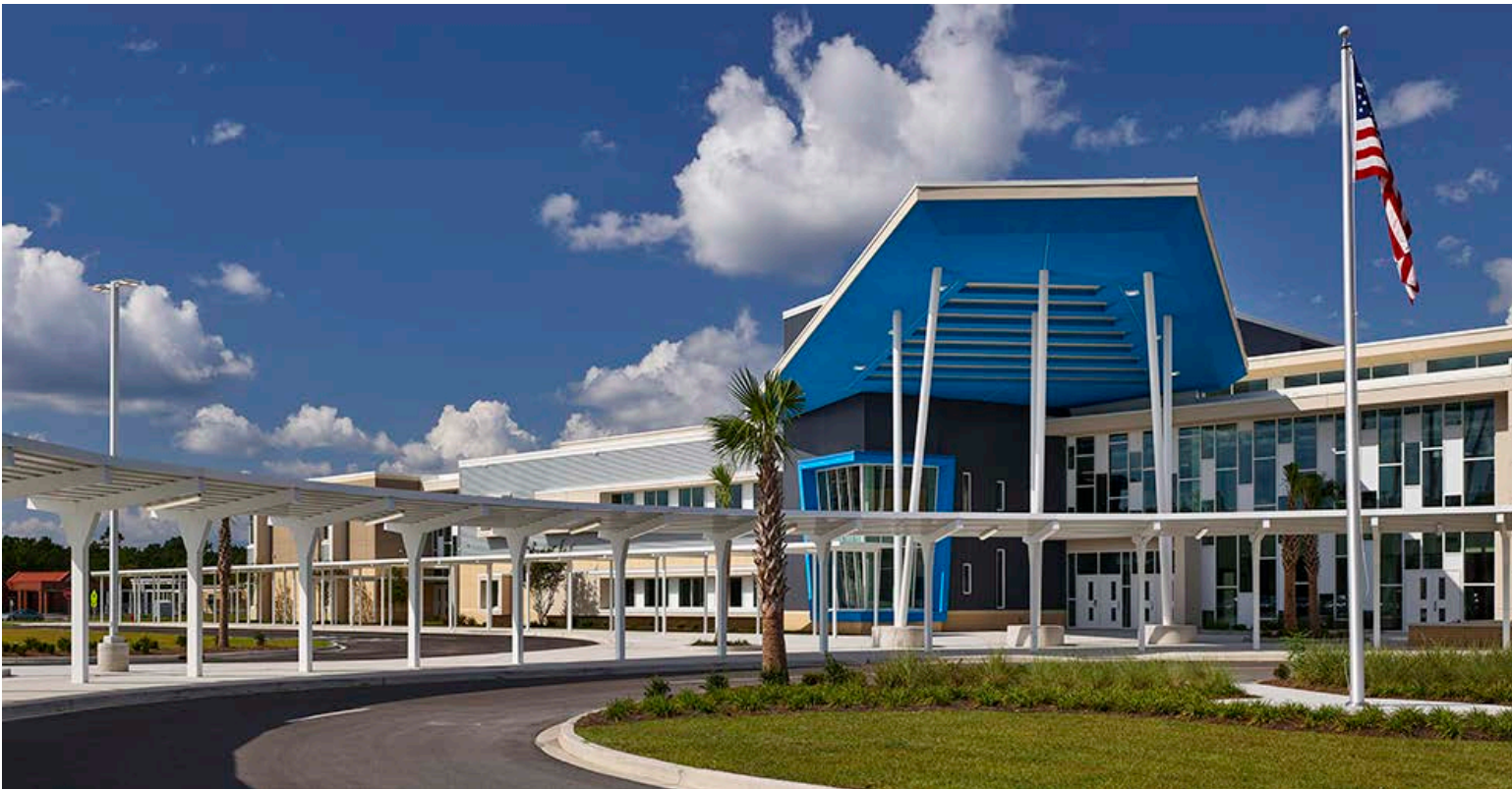
St. James Intermediate School in Myrtle Beach, South Carolina, which opened in August 2017, serves fifth and sixth grades and has a goal of producing 10% more energy than it uses. Photo by Horry County Schools
