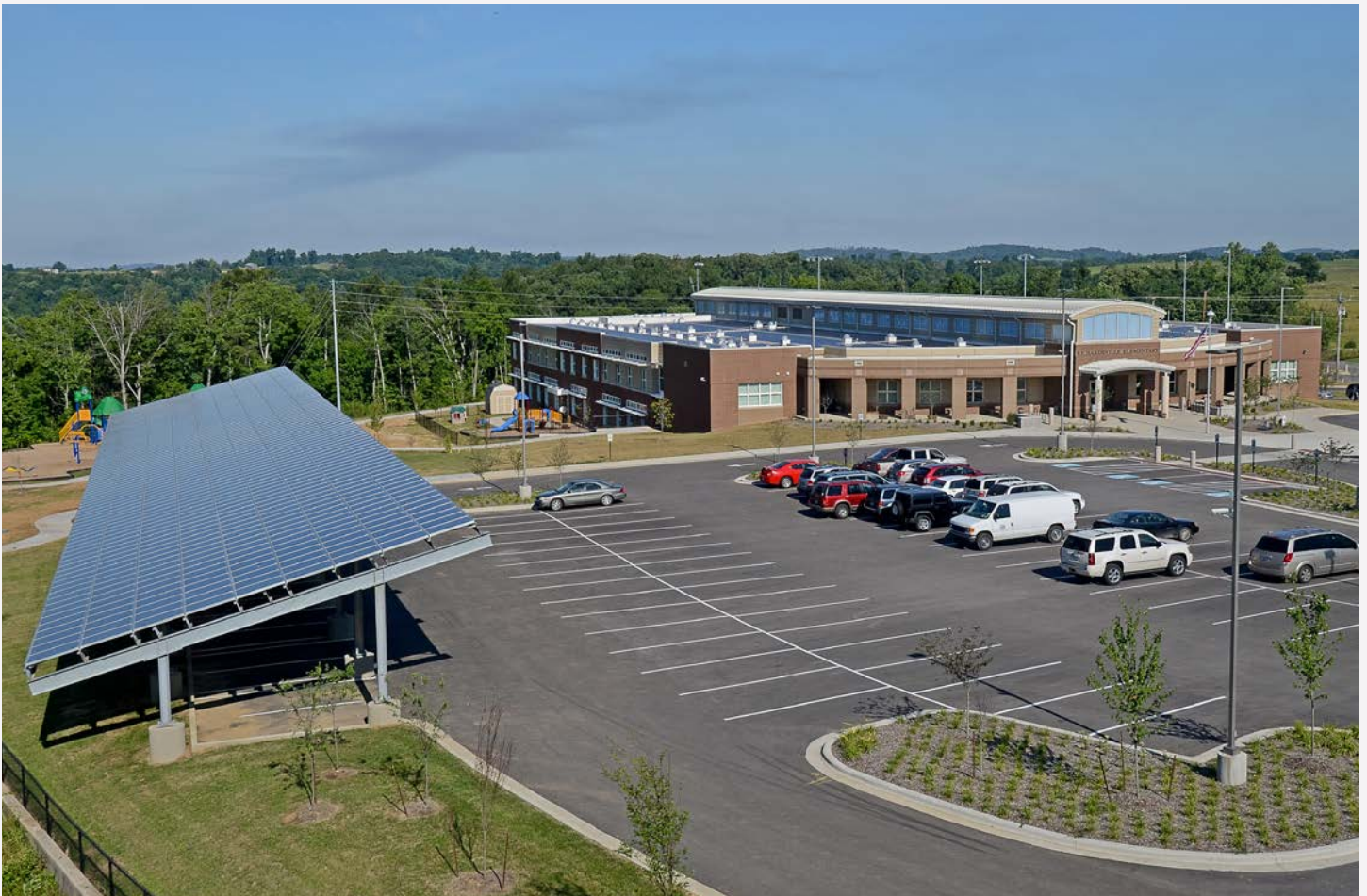
Richardsville Elementary, the first zero energy public school in the United States, operates at an EUI of \text{kBtu}/\text{ft}^2\text{-yr} , and produces more energy than it uses. The district receives an annual refund from the electric utility of more than $30,000 for the excess generation. Sherman Carter Barnhart Architects, Photo by Joshua White
