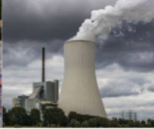
Factory steam Tower
