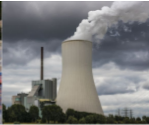
Factory steam Tower
